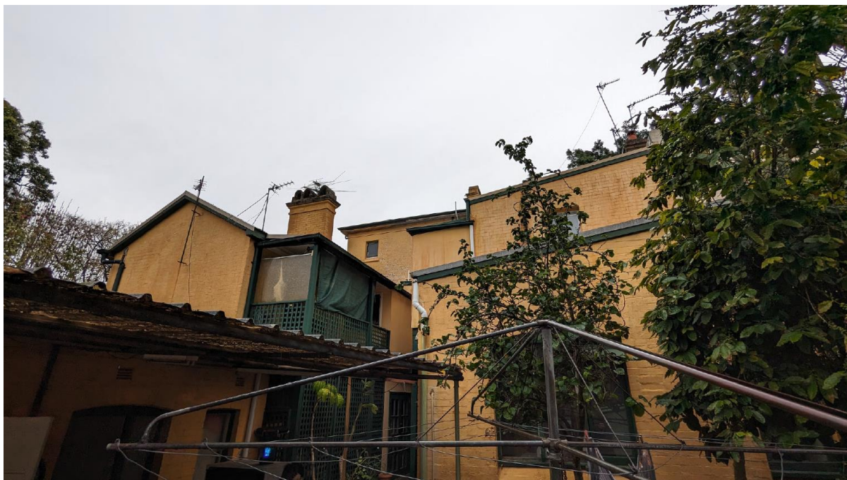
Figure 10: Rear elevation of 62-64 Selwyn Street
